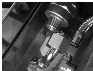
Connecting the metal hose
